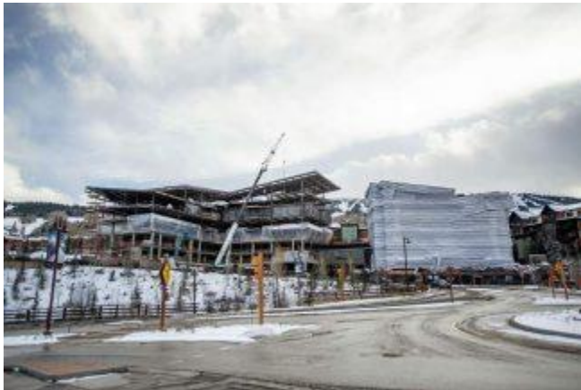
Base Village construction on Nov. 23. Buildings 7 and 8 are scheduled to open in 2019.
