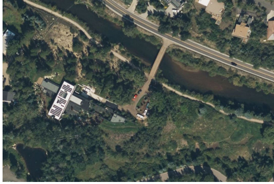
Accessed by a bridge over the Roaring Fork River, the property is about 4.23 acres. PHOTO: EAGLEVIEW
