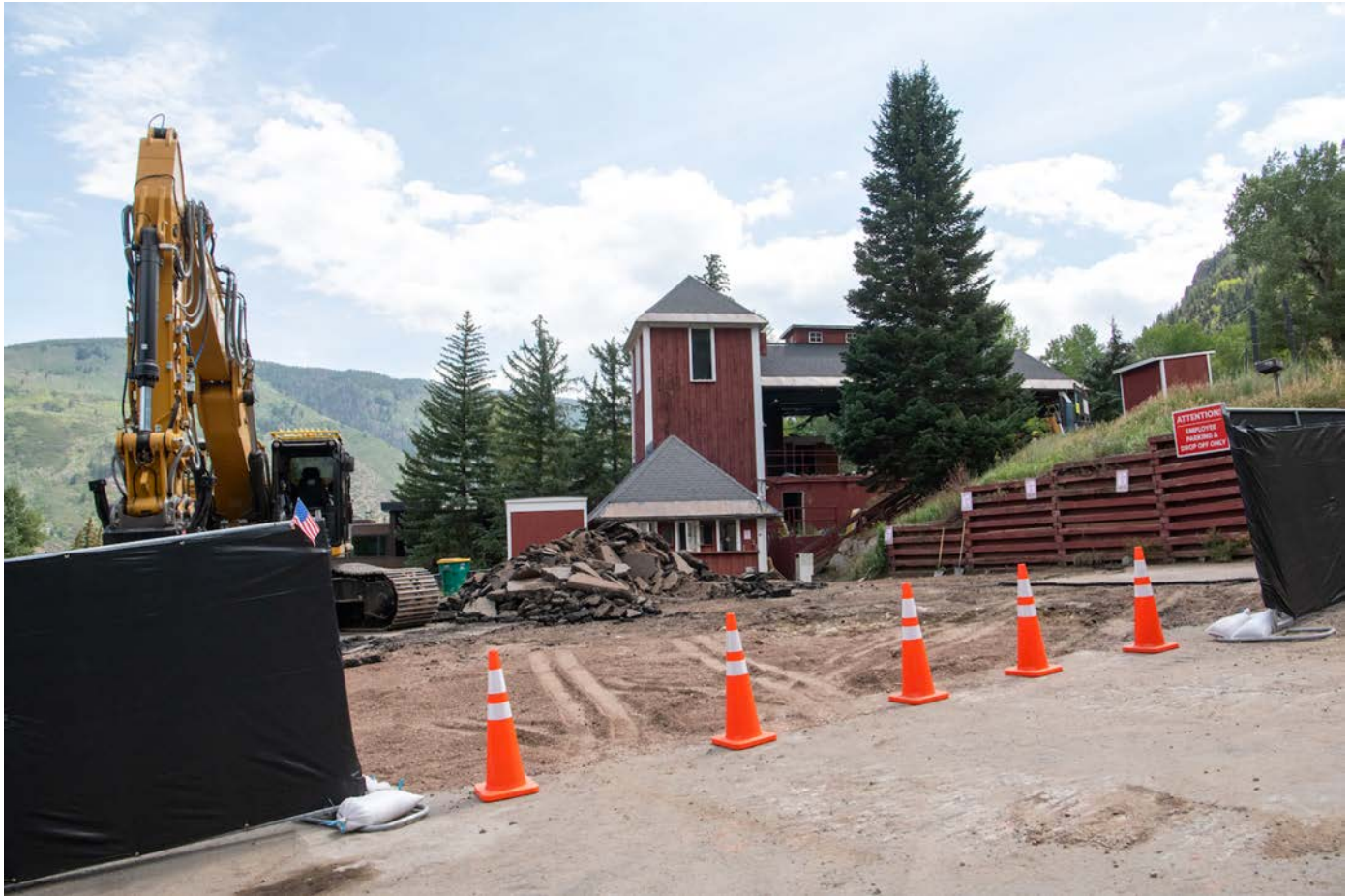
Cones and construction equipment sit at the base of Aspen Mountain's Lift 1A, also known as the Shadow Mountain lift, on Wednesday. Work to remove the lift is already underway as crews prepare for a major redevelopment of the Lift One corridor; the red building pictured here will be demolished to make way for the project, while some older historic assets will be relocated and restored. Jason Charme/Aspen Daily News
