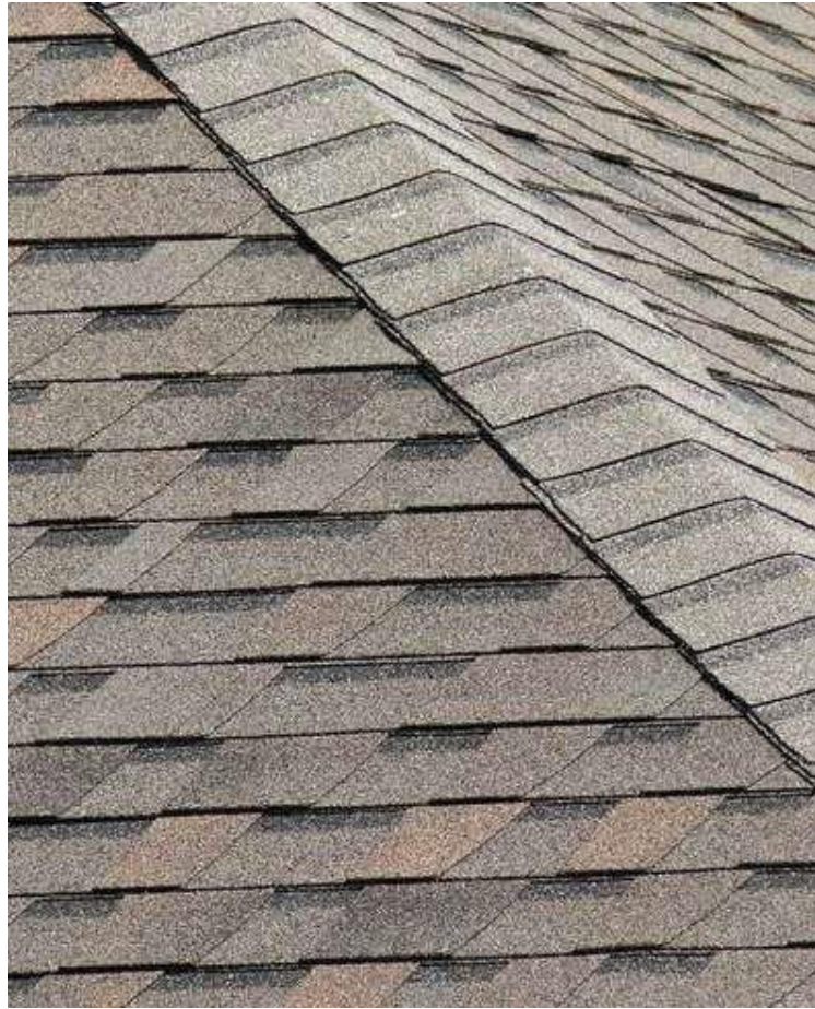
EXISTING ROOF MATERIAL ASPHALT SHINGLE
