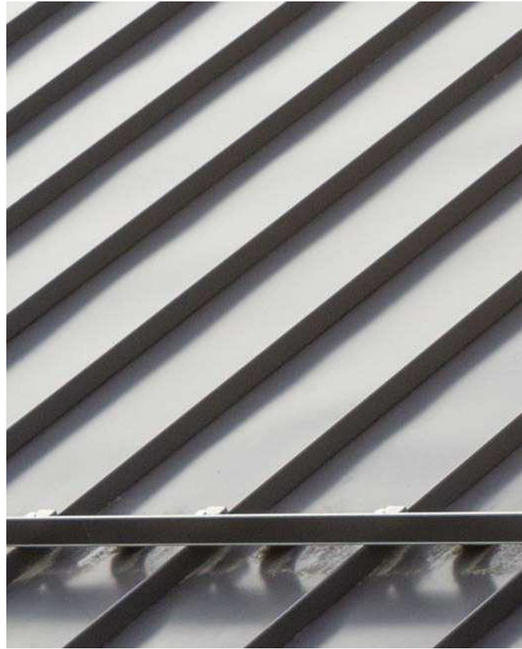
PROPOSED ROOF MATERIAL - A STANDING METAL SEAM
